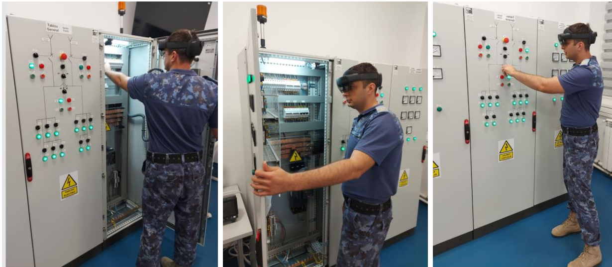
Figure 3. AR in marine power plant education and training
